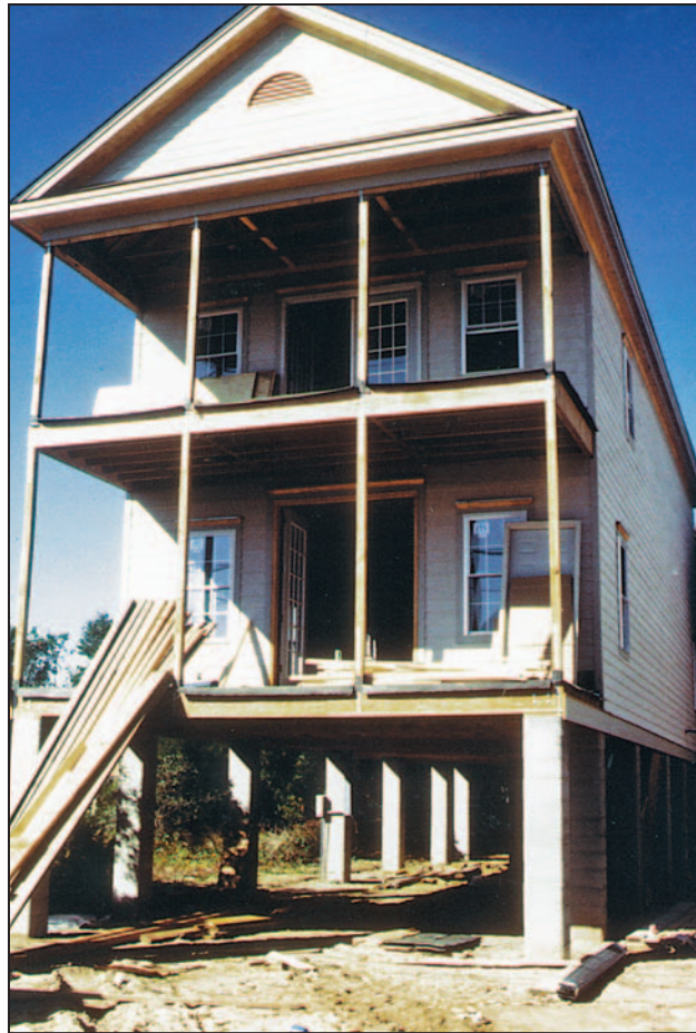
Figure 13-6. Open masonry foundation
